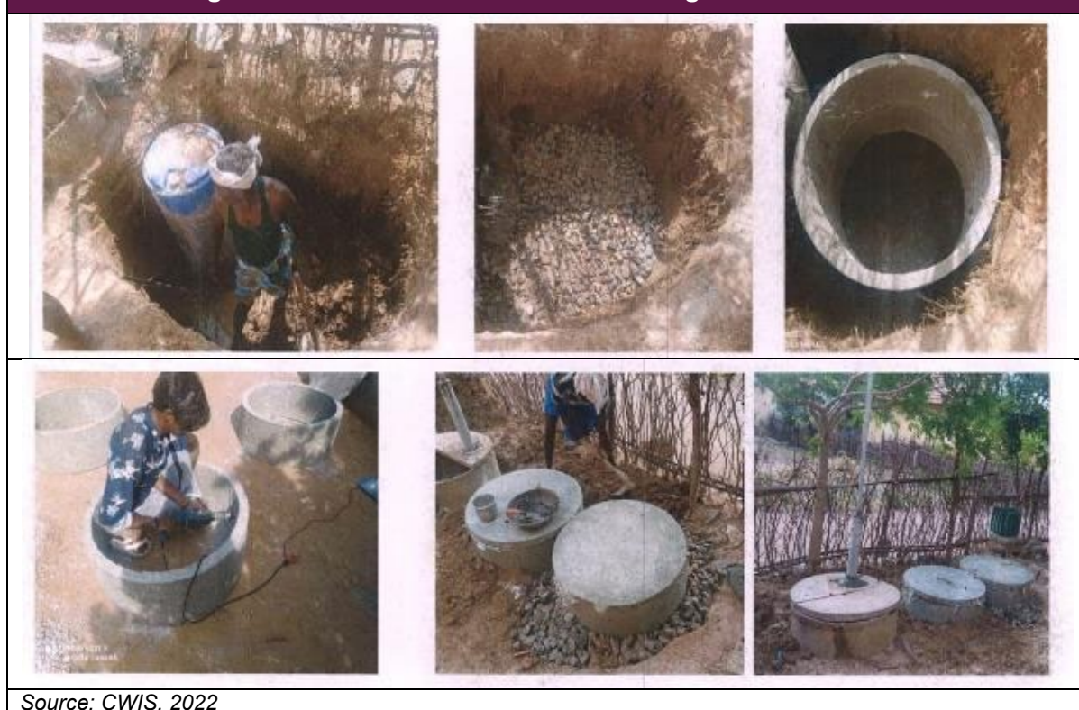
Figure A5.3: Installation of DRDO Bio Digester for Twin Pit
