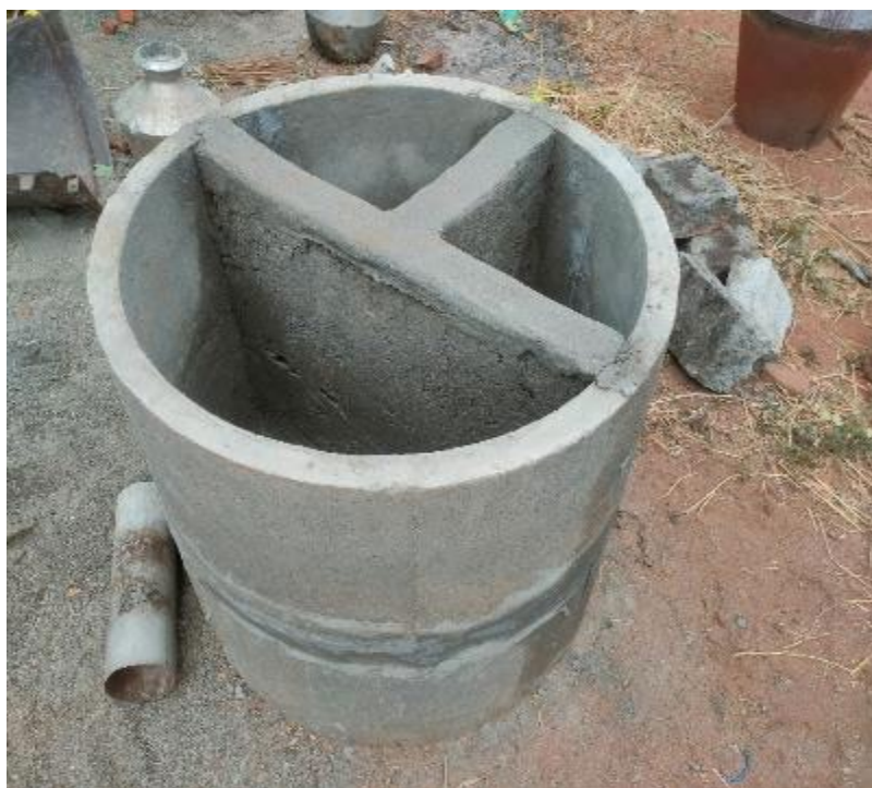
Figure A5.2: Reinforced Cement Concrete (RCC) Biodigester
