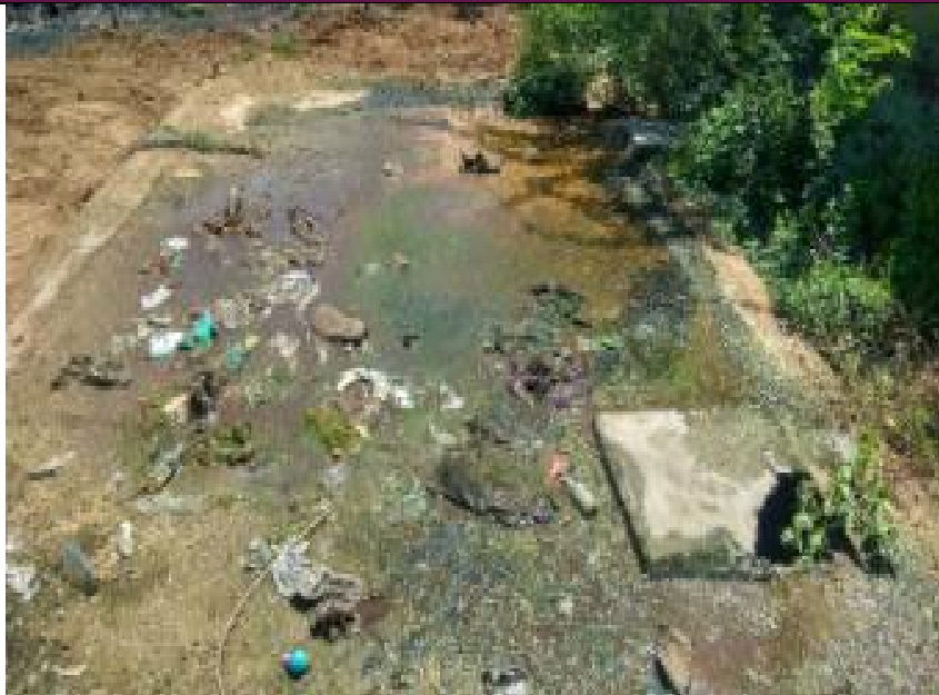
Figure 3.7: Status of containment before intervention in Thulasinganagar
