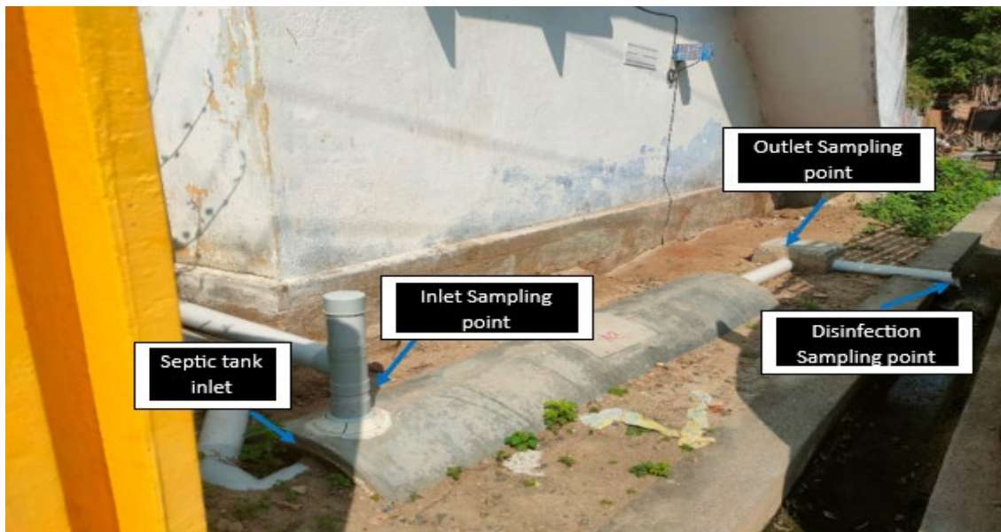
Figure A2.4: Sampling Points for RCC prefabricated septic tank
