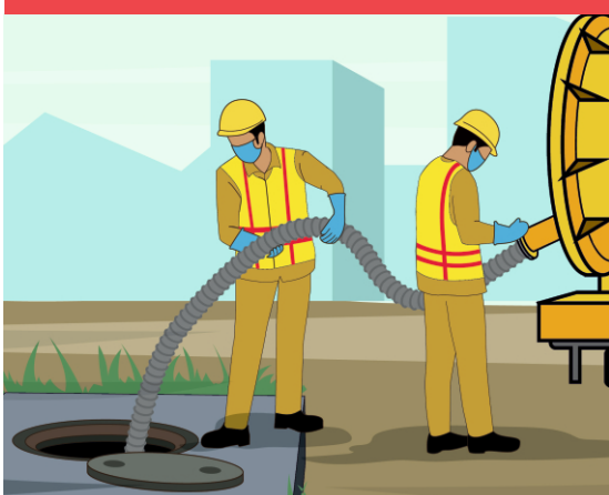
Figure 8: Emptying Septic Tank
