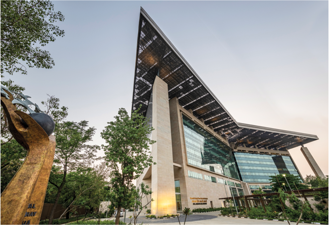
Atal Akshay Urja Bhawan, New Delhi. Source: Edifice Consultants Pvt. Ltd.
