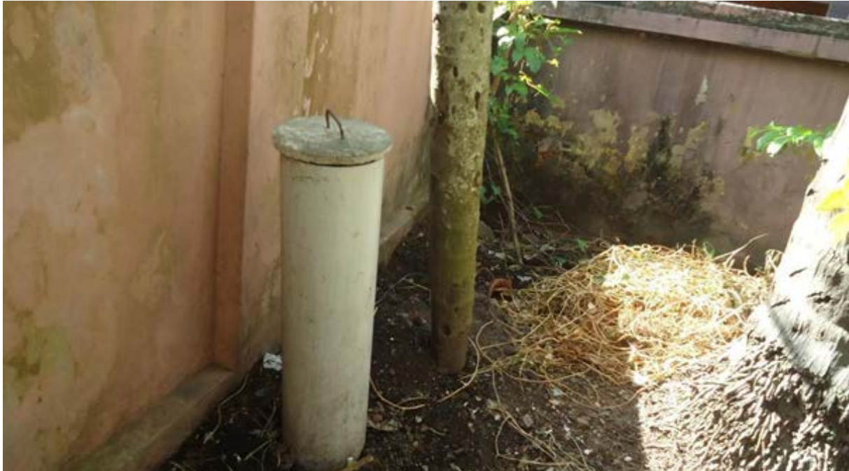
Figure 29.2: Pipe compost unit in a household in Thiruvananthapuram Source: Anita Pinheiro
