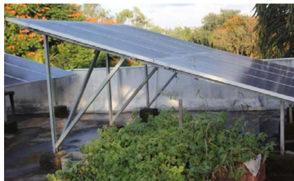
Figure 8.1: Roofs as multifunctional spaces—solar panels, rainwater harvesting, and vegetables all find place in PMC's Ghole Road office rooftop Source: Maitreyi Koduganti, September 2021
