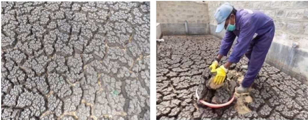
Figure 4.6: Dry sludge condition before removal from bed & removal of dried sludge
