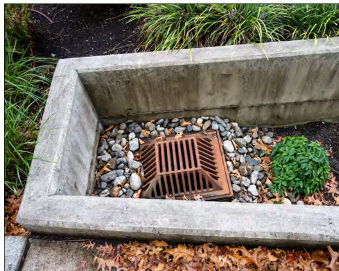
Bioswale, a channel that manages stormwater runoffs
